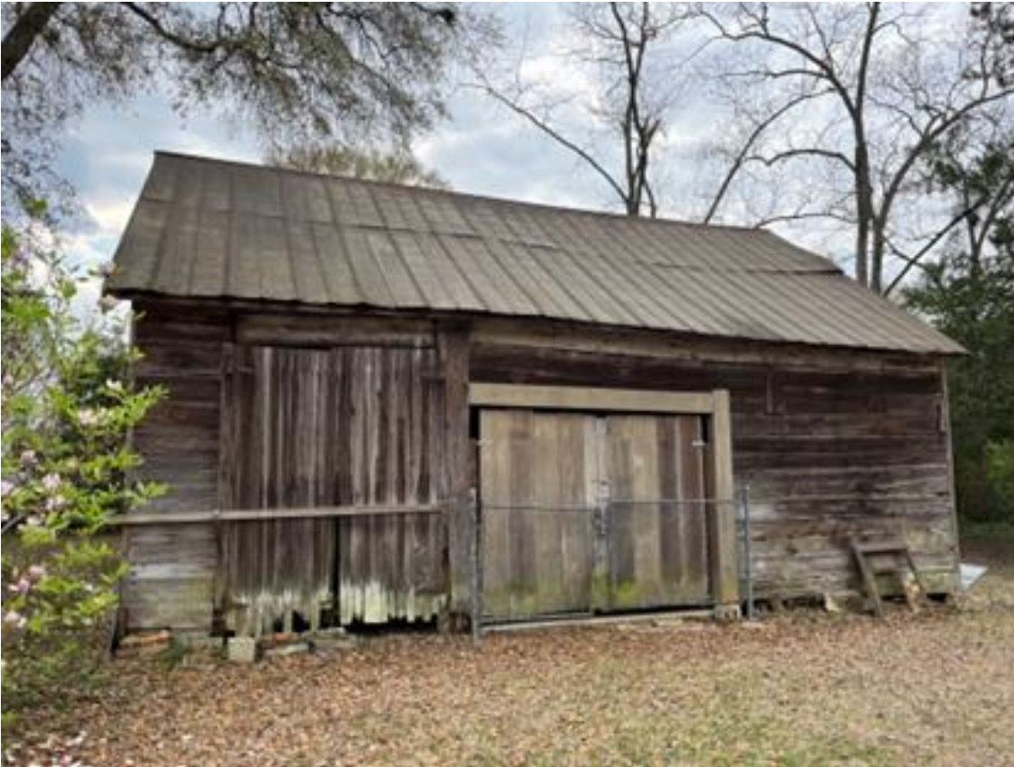
807 Washington Street Secondary Structure
