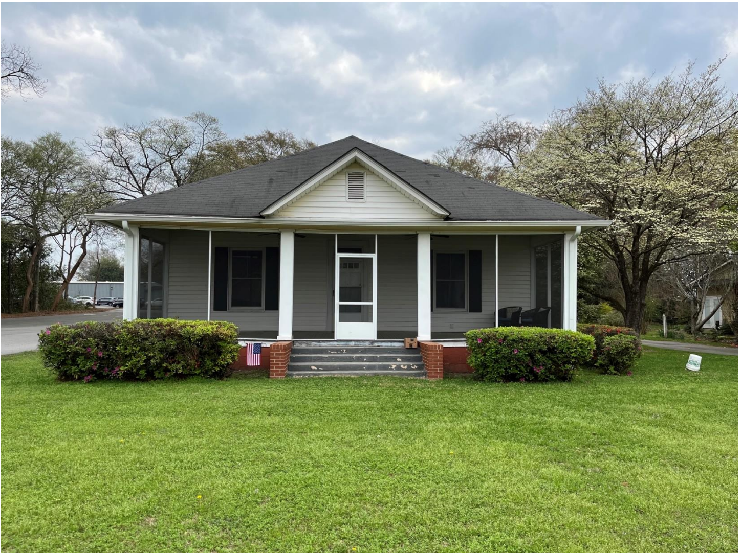
/Hull House 1920 No Academic Style Rear addition
