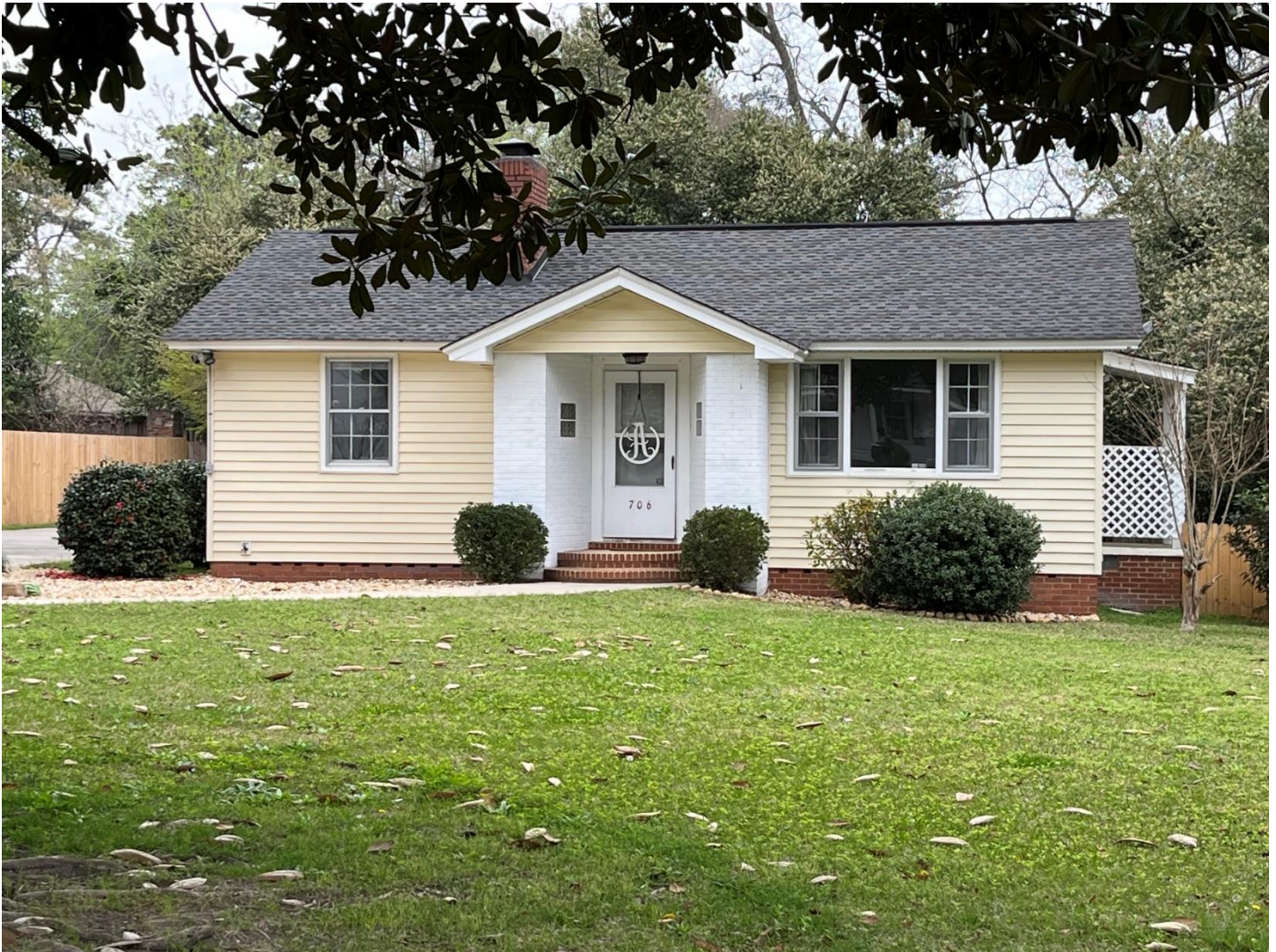
/Anderson House 1946 No Academic Style Rear addition Vinyl siding
