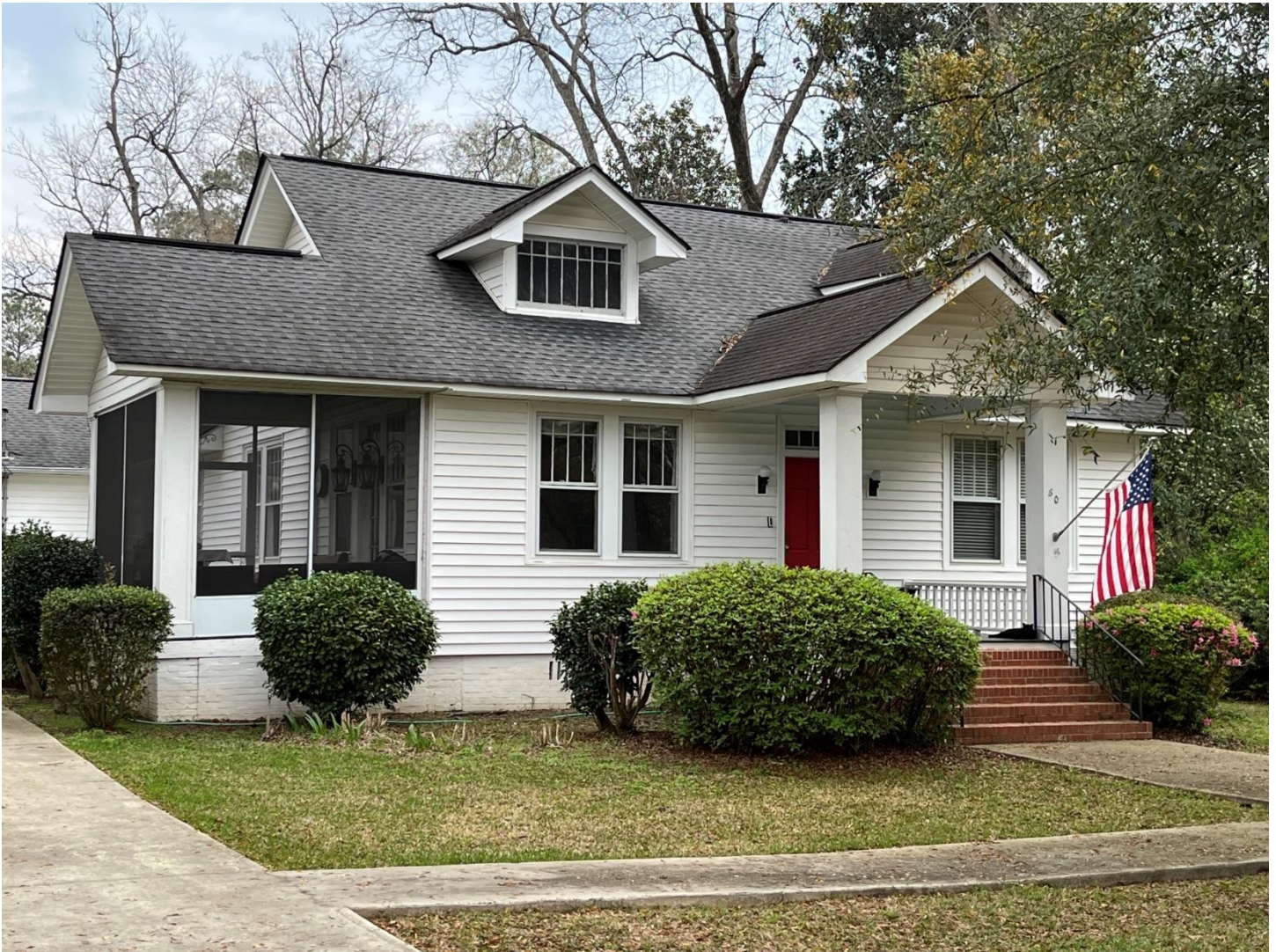
/Overton House 1925 Craftsman Vinyl siding, rear addition
