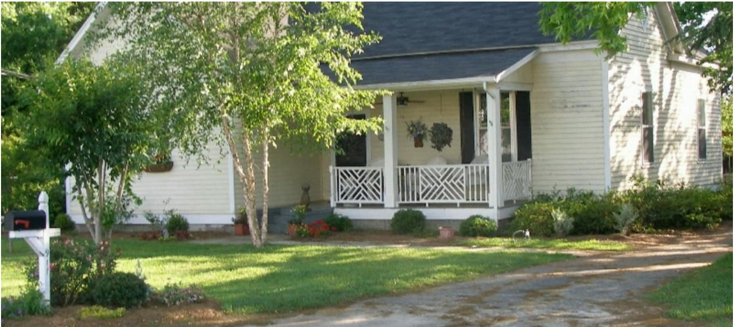
Anderson House/rental c. 1900 Folk Victorian Altered window size, vinyl siding
