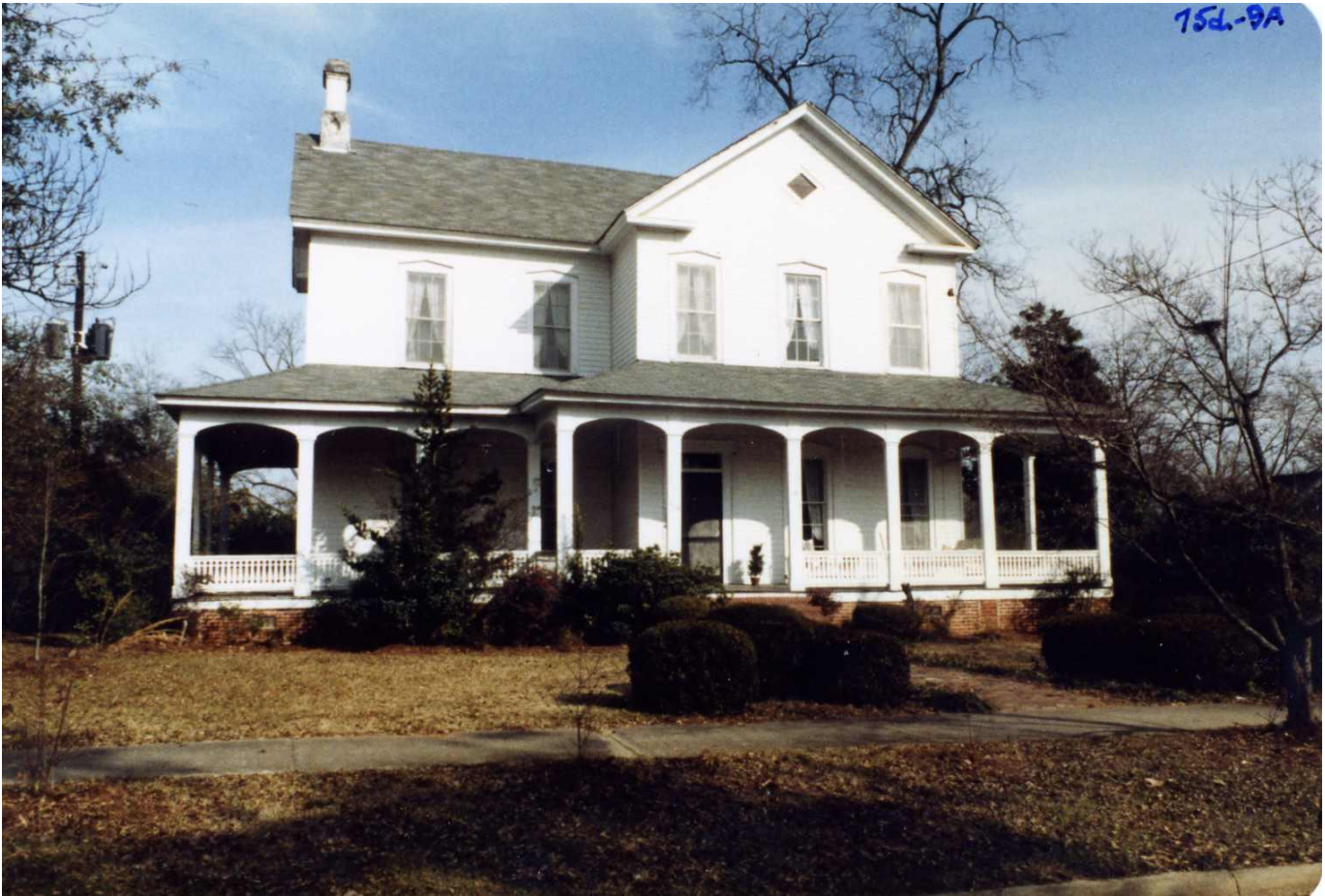
Pringle House/James House
